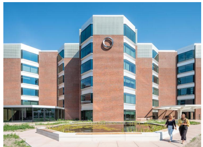
Water body at Entrance
