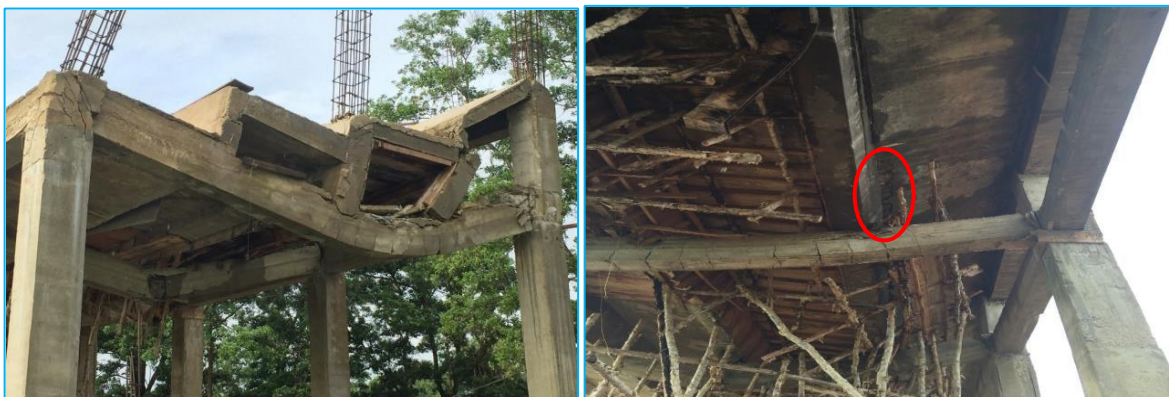
Figure 1. Structure of concrete beams and floor slabs-1
