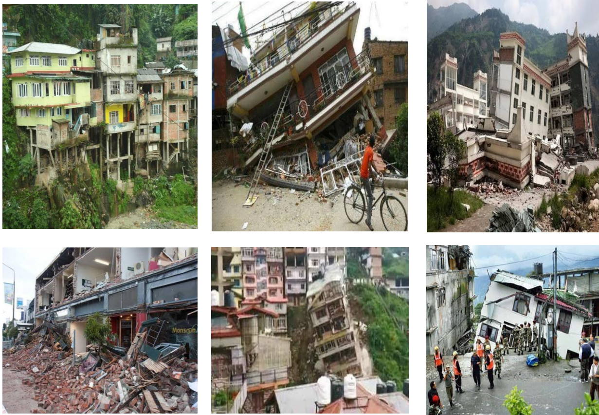
Fig. 1. Damage and collapse of buildings due to earthquake in hilly areas.
