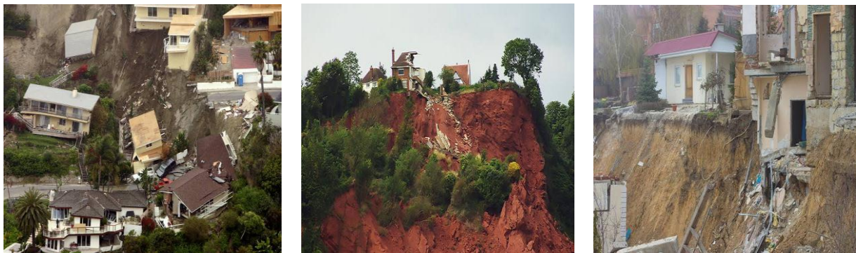
Fig. 4. Collapse of buildings due to land slide.
