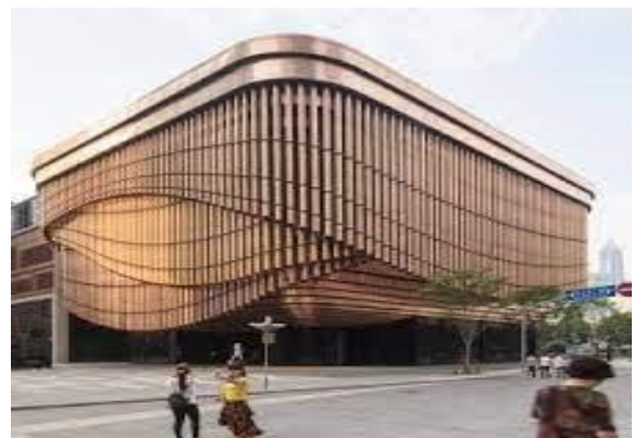
Fig 3: view of the building
