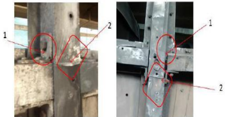
Fig -2: Pillars break near joints
