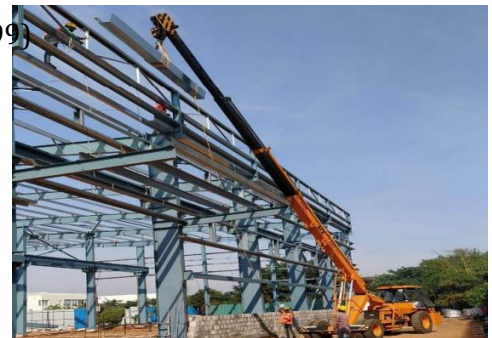
Figure 4: Gutter Installation work at site:
