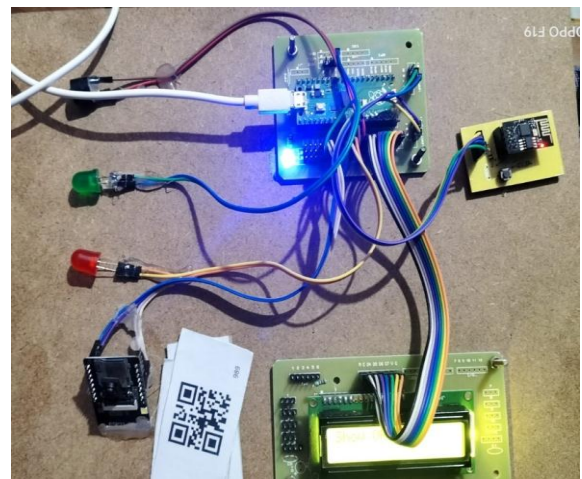
Fig 5: Circuit Implementation after Power supply Turn on
