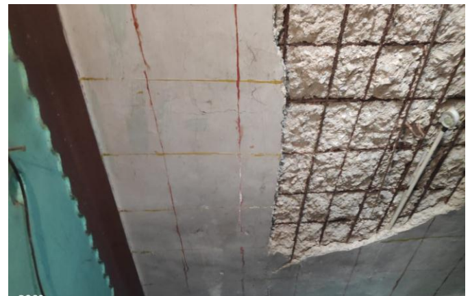
Figure 5.1: Grid pattern on the ceiling
