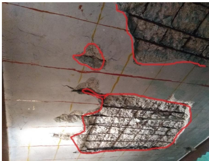
Figure 6.2: Weak Compressive strength zone
