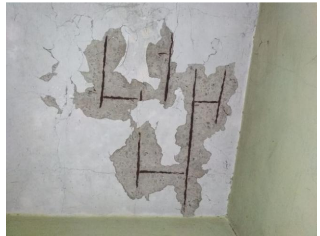
Figure 4.2 : Damaged Slab
