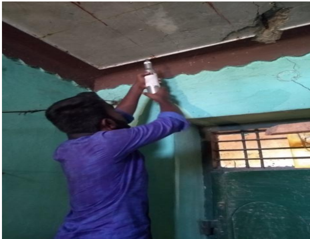
Figure 5.3: Rebound Hammer Test
