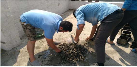
Mixing of concrete
