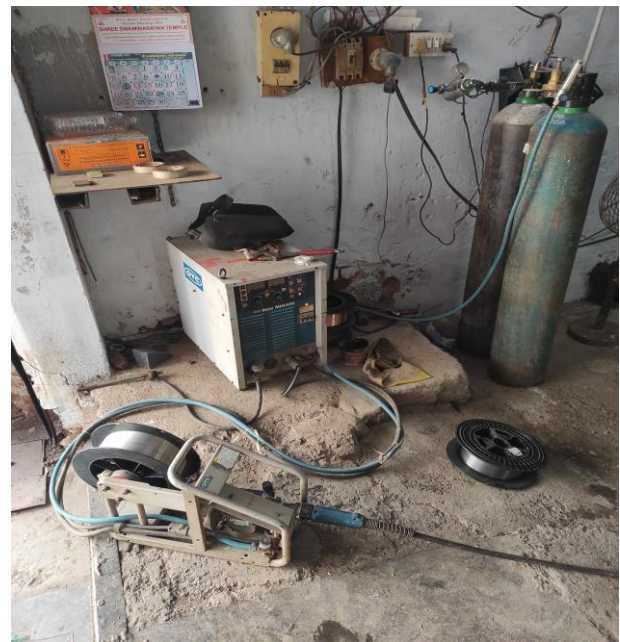
Fig-1: MIG Welding Machine set-up
