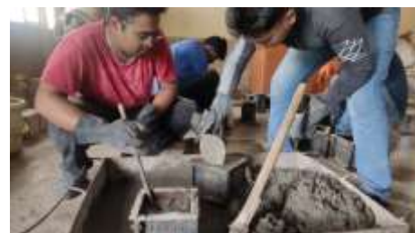
Fig.9 Placing and compacting the freshly concrete in moulds
